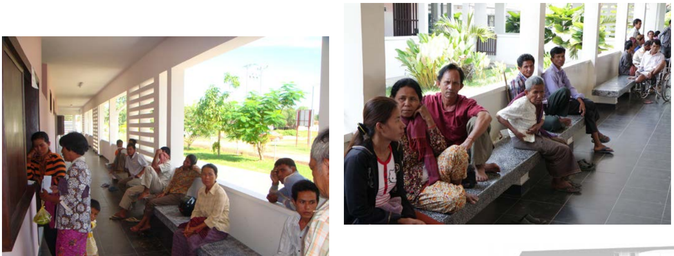
Figure 3: Open, airy verandahs allow for air movement, keeping the hospital cooler, and creating a pleasant environment for patients to wait. ©CTEH
