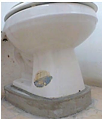
Photo 7: Raised toilet seat with concrete base
