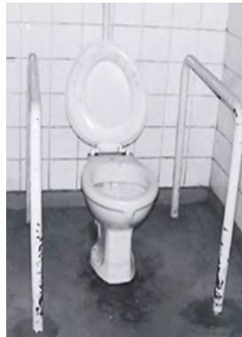
Photos 4, 5 and 6: Various examples of grab bars installed by the toilet
