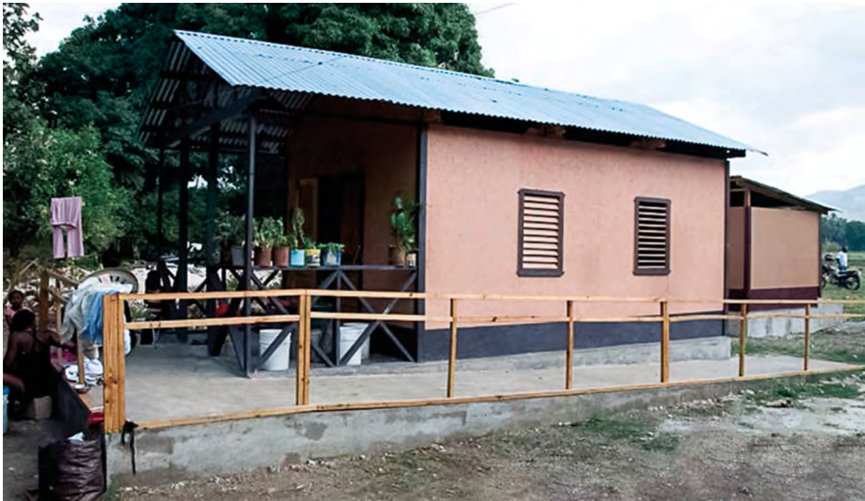
Photo 1: Accessible shelter with access ramp (gradient 1:20)
