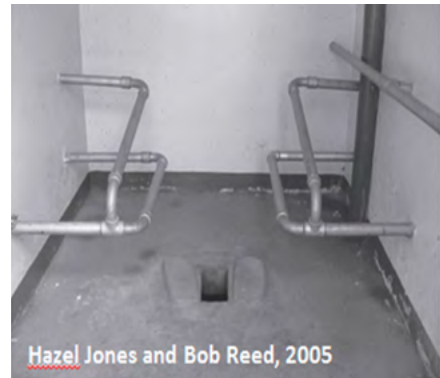
Photos 4, 5 and 6: Various examples of grab bars installed by the toilet
