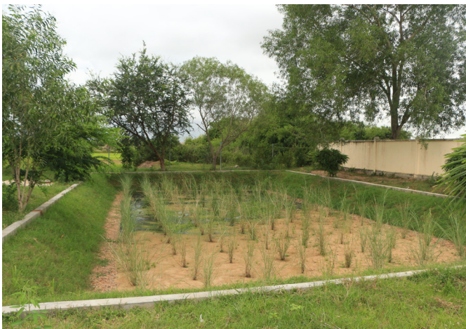
Figure 10: In order to protect local waterways and villages from hospital sewage and run-off water, a well designed sewage system has been constructed. This includes establishment of reed-bed pond. Fish have been added to eat mosquito larvae and other insects. Hospital staff use the area alongside the reed-bed to grow vegetables. ©CTEH/CBM
