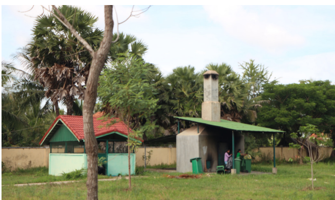
Figure 9: An incinerator in a locked compound ensures safe disposal of hospital waste, with minimal environmental risks and hazards to the local population. ©CTEH/CBM
